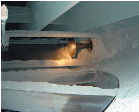
Installation from the inside of the Air heater
