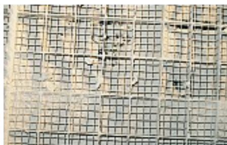
SCR, after six months process without Sonic Cleaning
