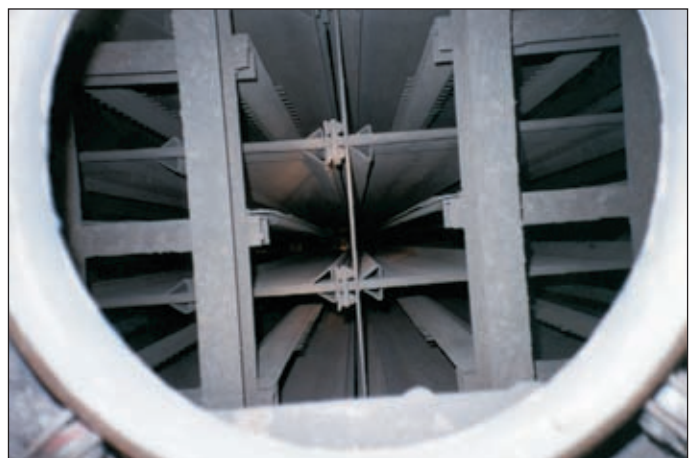
After six weeks production with Sonic Cleaning. Dust emission 13.5\text{mg}/\text{Sm}^3
