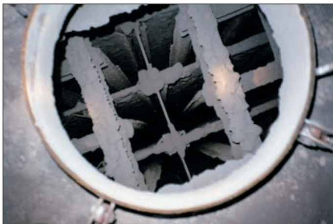
After six weeks production without Sonic Cleaning. Dust emission 29.4\text{mg}/\text{Sm}^3
